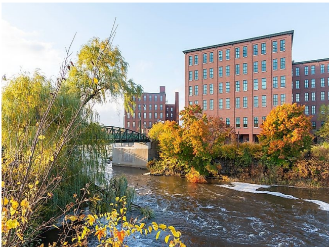
RENOVATED MILL BUILDING IN DOWNTOWN WESTBROOK
